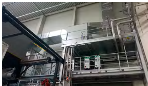
The exhaust air filter and the exhaust air ducts can also be mounted next to the casting machine to save space.
